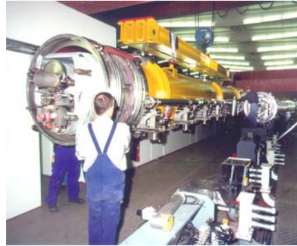
Installation of modules into the accelerator
