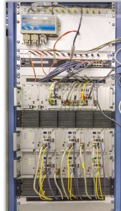
Retrofitting controls rack controlling power supplies
