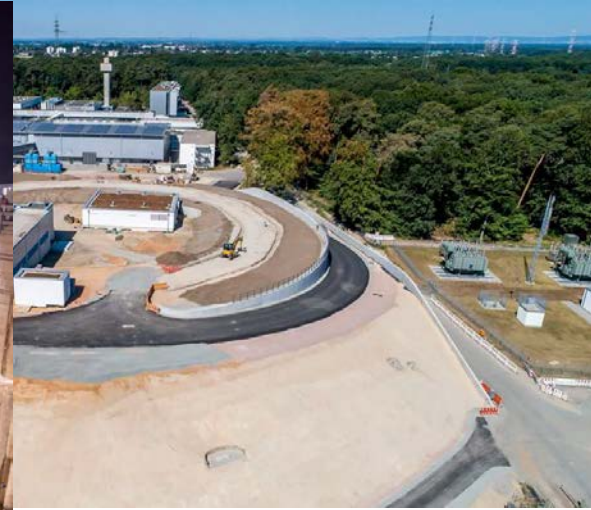
Completed ready for FAIR and FAIR phase 0
