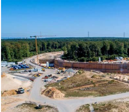
Excavation SIS100 tunnel
