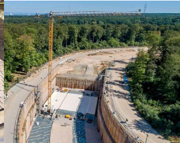
Start of concrete shell works for SIS100
