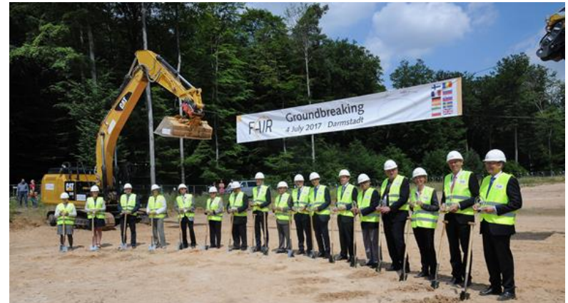
Ground breaking - 4 July 2017
