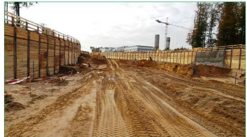
Excavation SIS100 tunnel - Nov 2017
