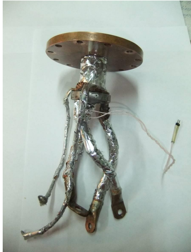
old transfer lines
