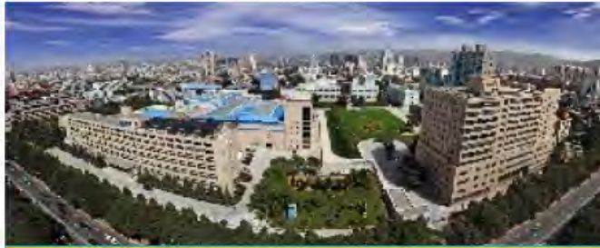
IMP main campus National Laboratory of Heavy Ion Accelerator in Lanzhou (NLHAL)
