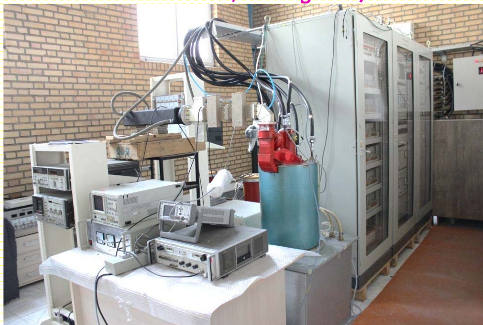
Linac laboratory at IPM, RF (klystron, modulator, waveguide)
