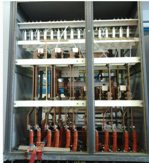
New power-cable laying and connection in June 2015
