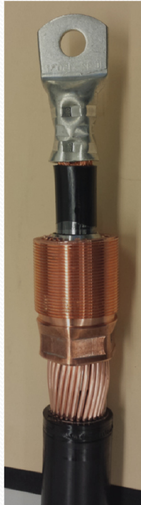
Copper bushing fixed over the outer conductors
