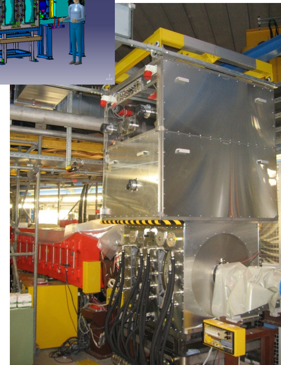
Installation of first module completed, tested with beam.
