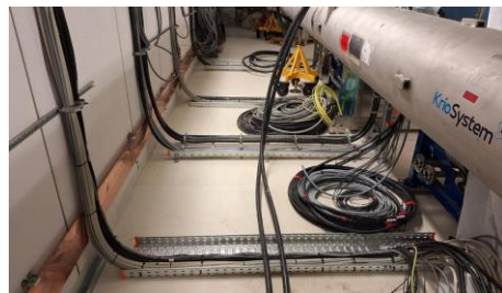
Machine trays and cable end laying
