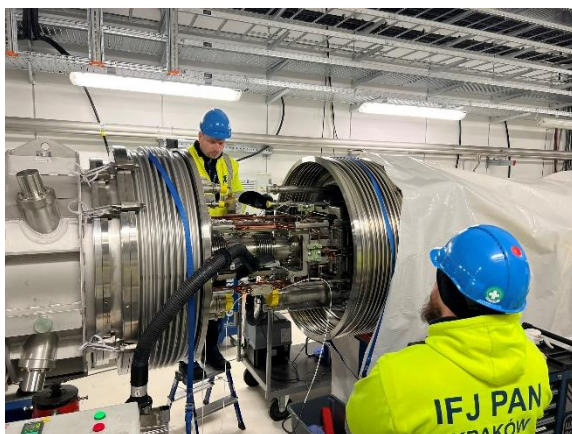
IFJ PAN brazes the busbars to the SIS100 module interconnections
