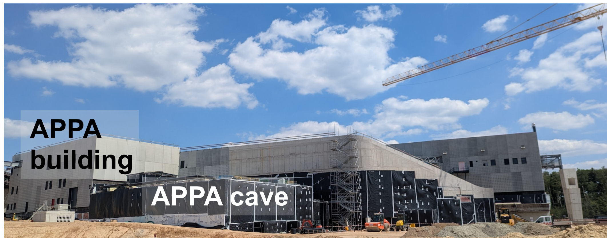
FAIR Construction Site, July 2026
