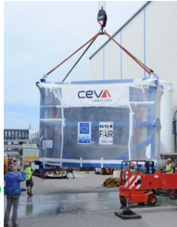
Whole OT in transport frame, 7x5.5x3.5 m 3 , 24t, arrival at GSI, Aug. 25, '23. (Photo courtesy: GSI)
