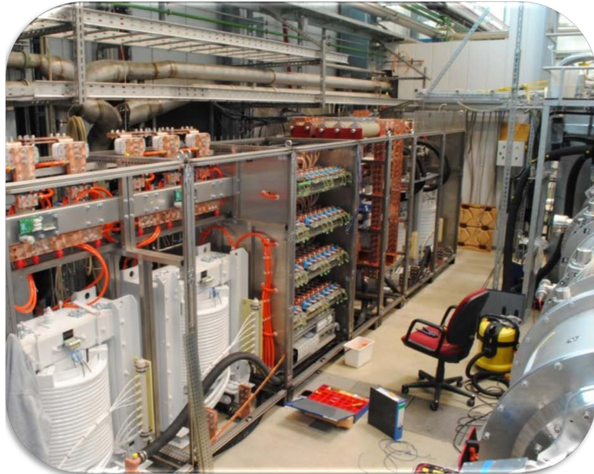
Power converter during assembly
