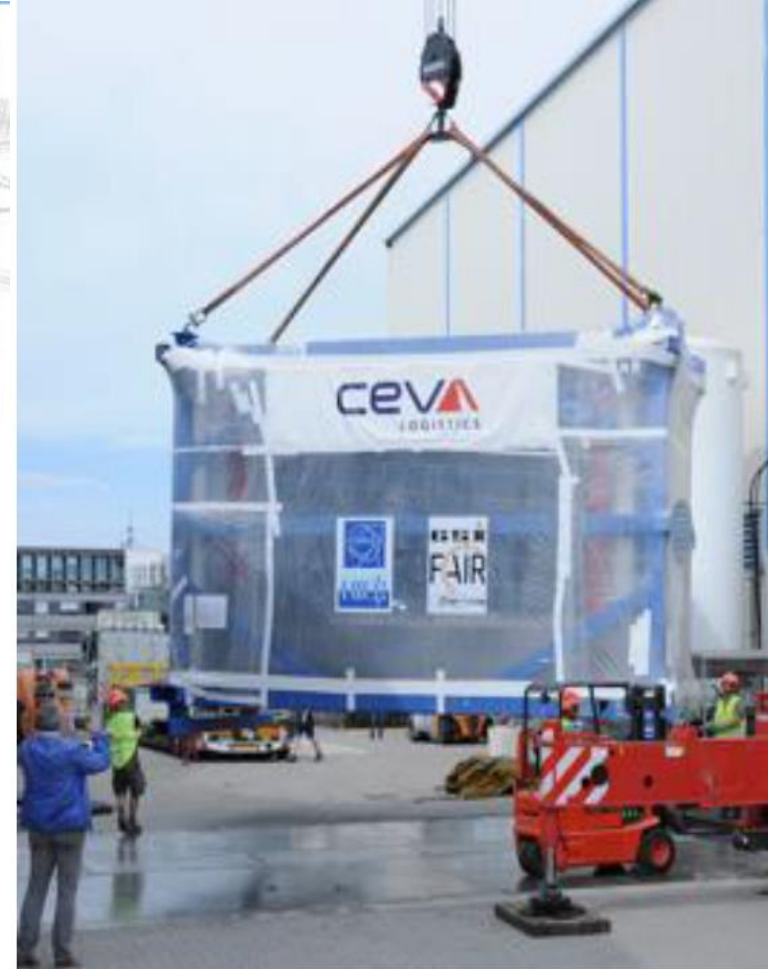
Whole OT in transport frame, 7x5.5x3.5 m 3 , 24t, arrival at GSI, Aug. 25, 2023. (Photo courtesy: GSI)
