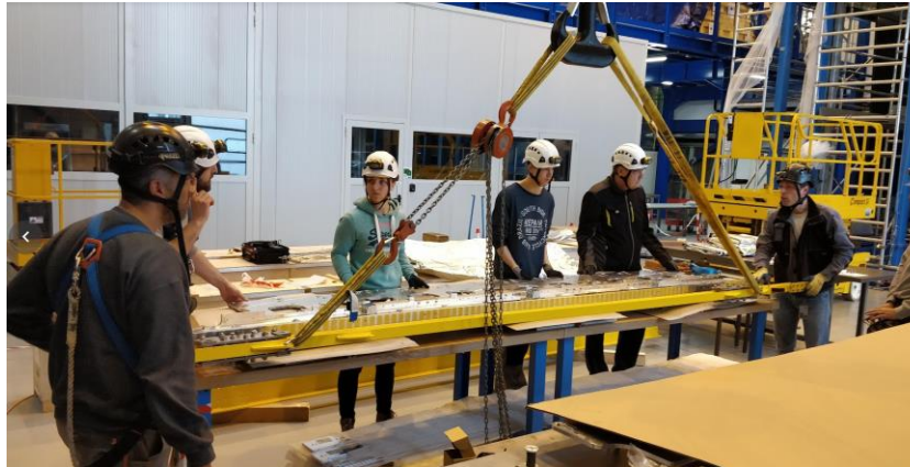
Assembling C-Frame mechanics.
