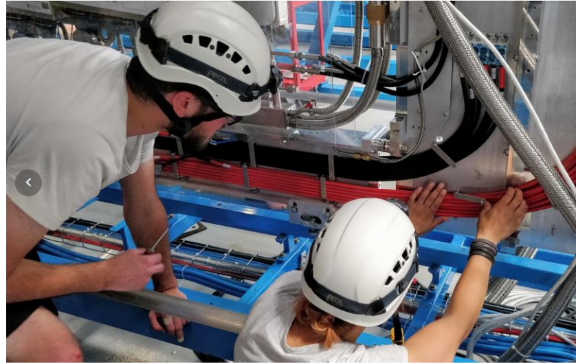
Installing bias cables.
