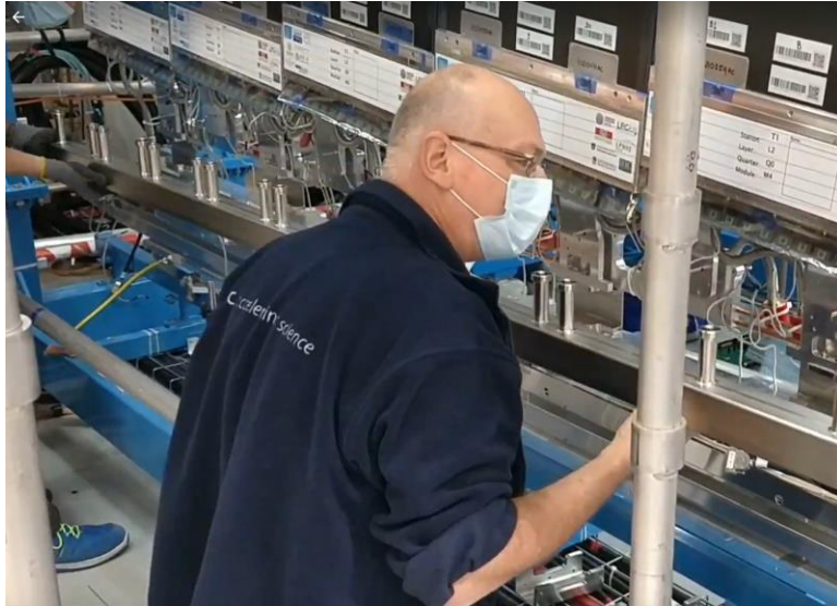
Replacing a defective cooling and vacuum manifold.
