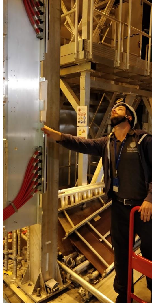
Testing installation of the mechanics.
