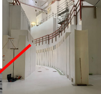
Target Area: installation of lateral iron shielding
