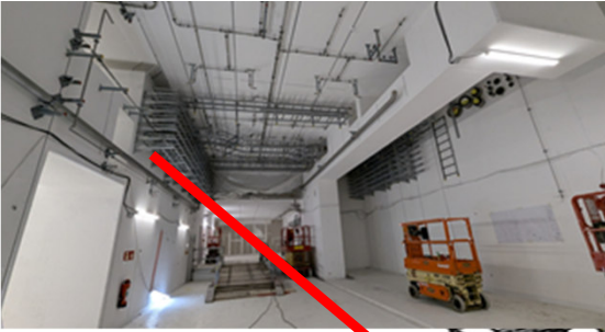
Pre-Target Area: installation of TBI advanced
