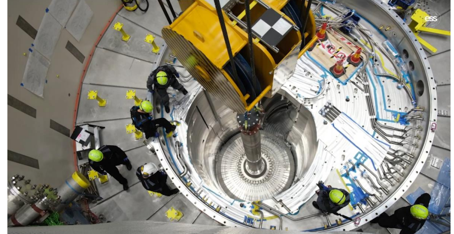
Target wheel installed
