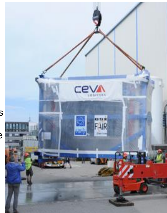
Whole OT in transport frame, 7 \times 5.5 \times 3.5 \text{ m}^3 , 24t, arrival at GSI, Aug. 25, '23. (Photo courtesy: GSI)
