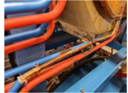
leak copper pipe..., brazed, ... insulated.
