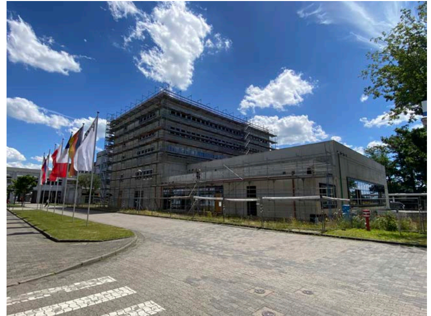
View of the north facade with the MCR
