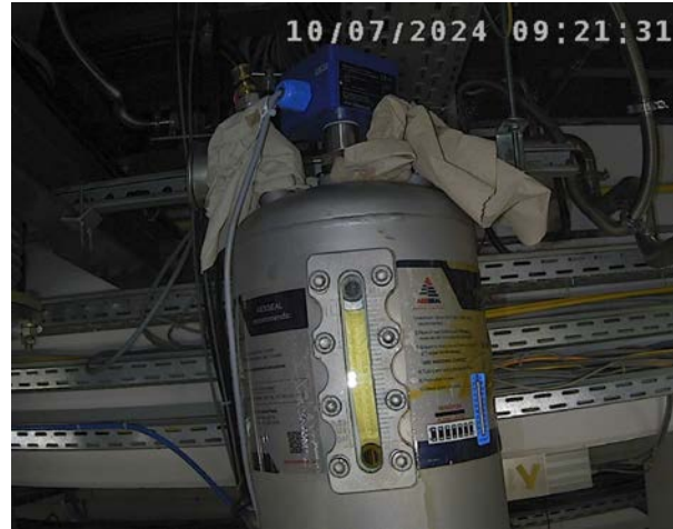
floating ring seal oil reservoir
