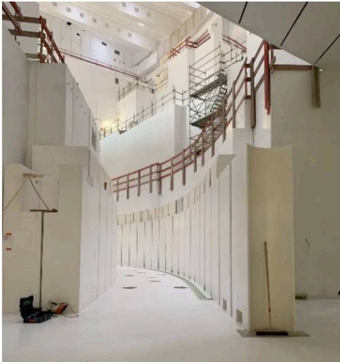
Installation of lateral iron shielding completed in July
