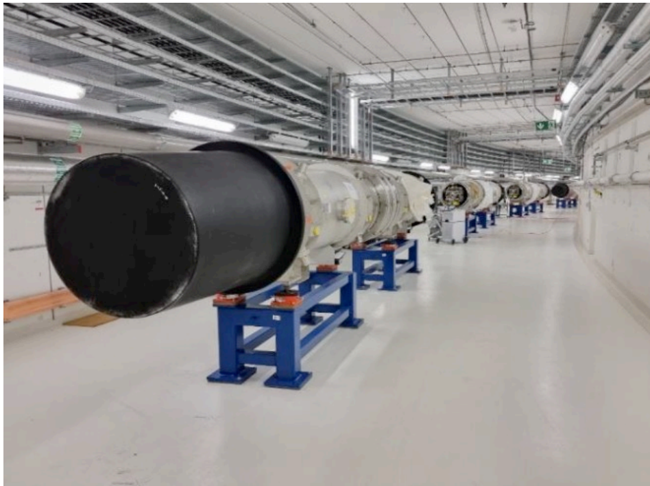
SIS100 Sector 3 Arc: Dipole Pairs Installation completed
