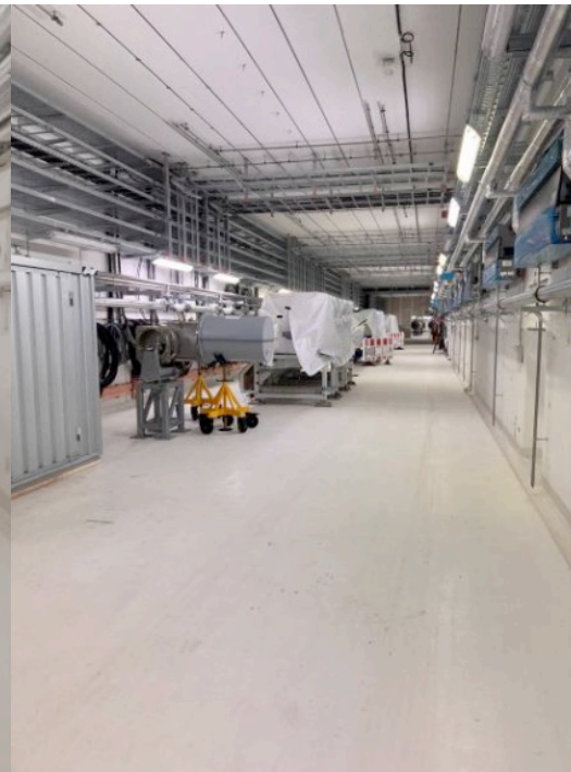
SIS100 Straight 4 – partially completed
