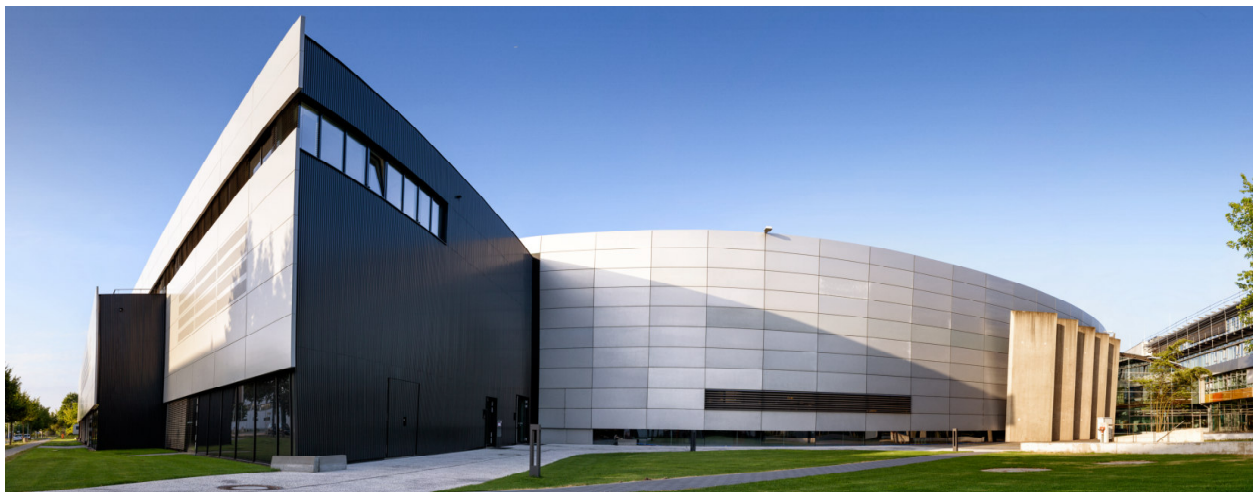
Figure 4: View of the BESSY II building
