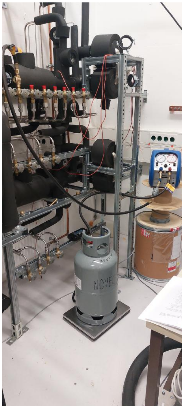
Figure 14: The drainage system connected to the cooling test rig
