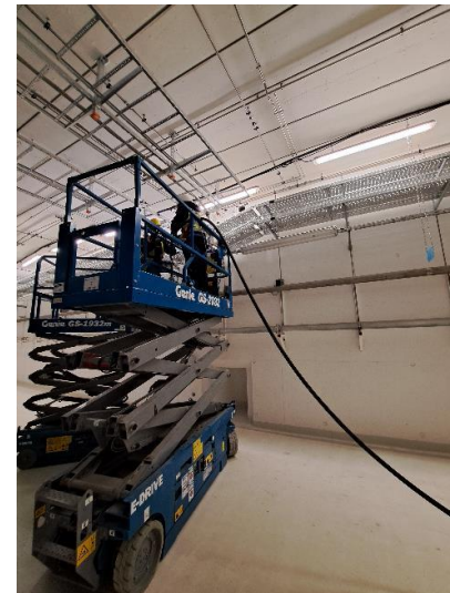
Preparatory cable pulling test was successfully carried out on 31.03.2023.
