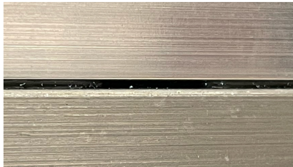
Figure 4.33: A hole in the epoxy grout between Aluminum frame (top) and distance ledge system (bottom) is shown.
