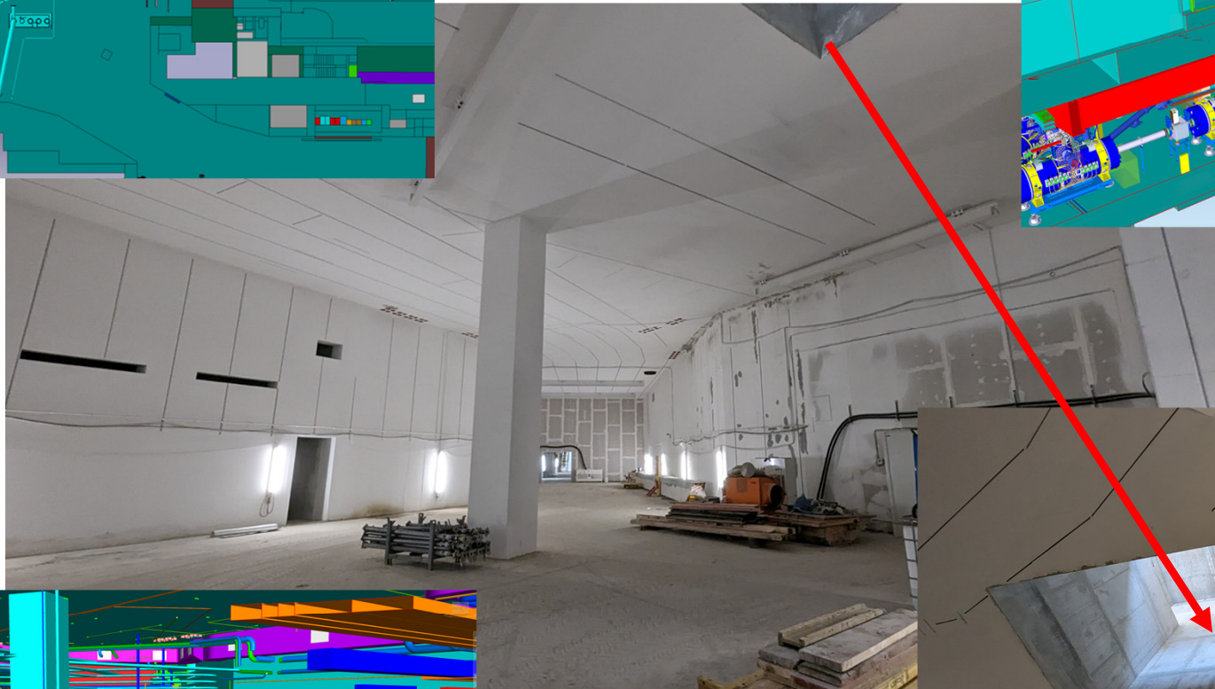
FHF1 roof opening (80 ton crane access)
