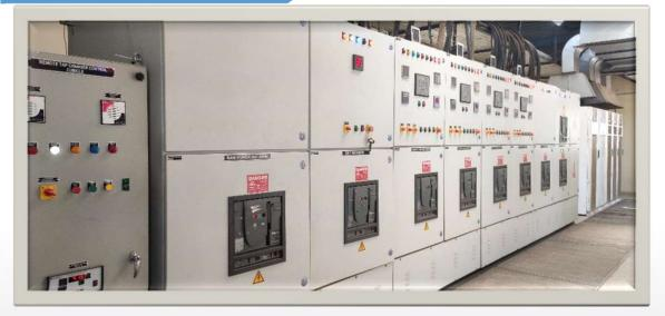
Entire plant under UPS of capacity of 1250 KVA and synchronized with 6 x Diesel generators of 2000 KVA
