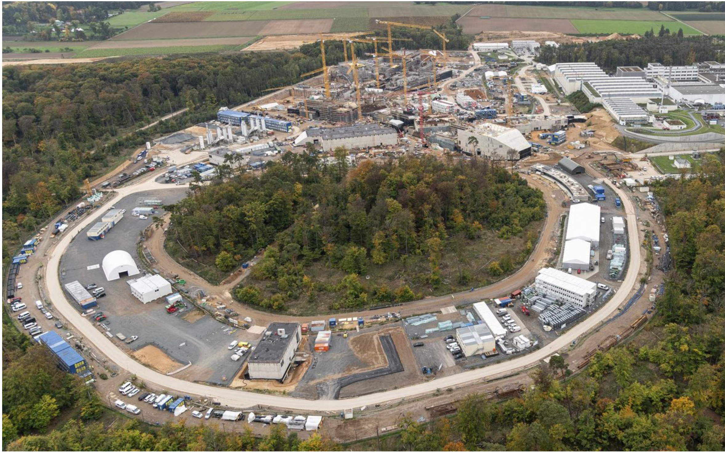
FAIR Construction Site, October 2022
