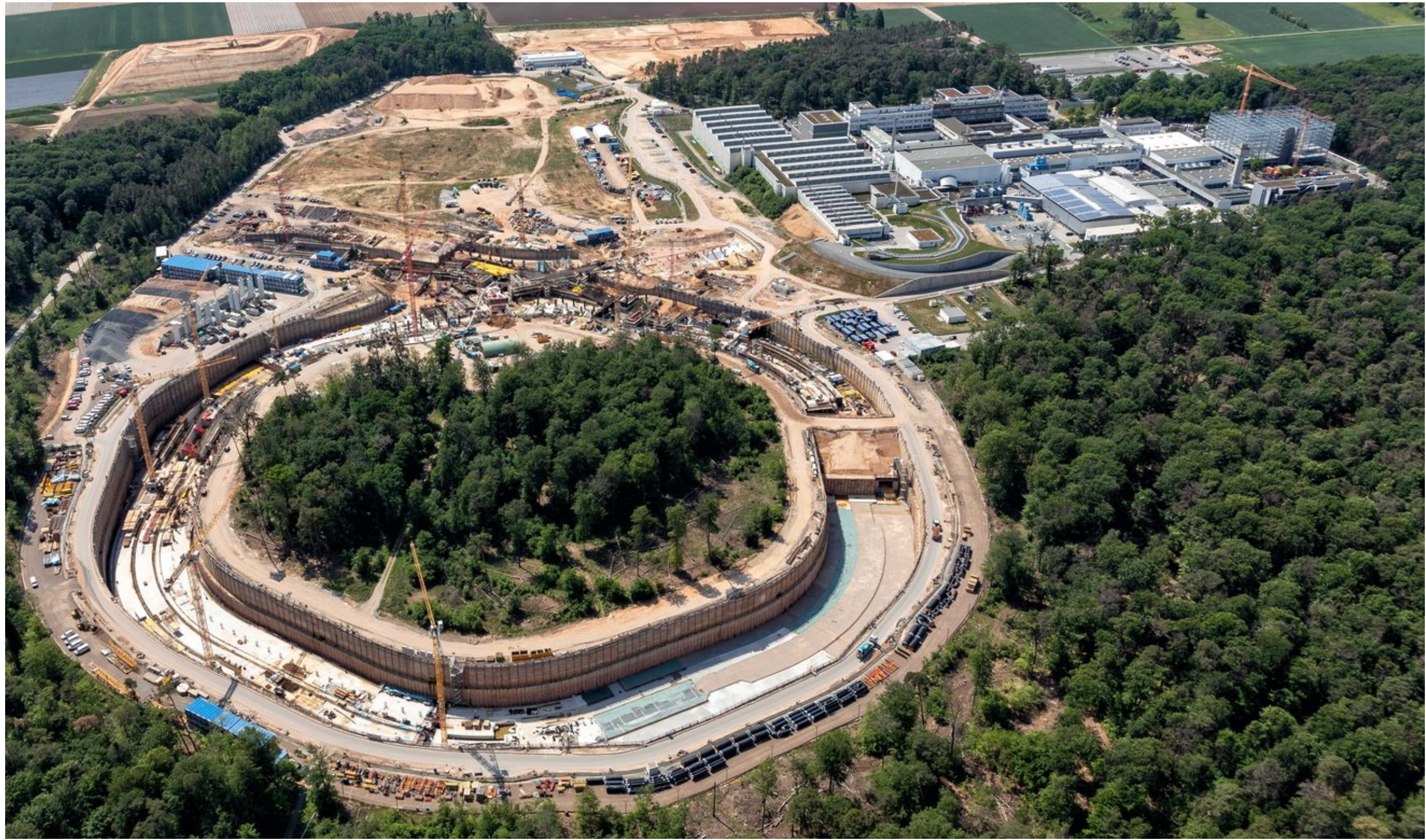
FAIR Construction Site, October 2020
