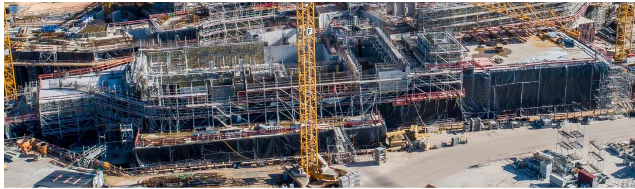
FAIR South Area Construction Site, October 2022
