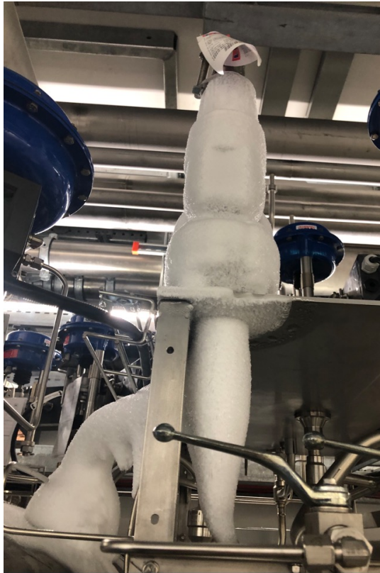
11 x SVs in 4.5K supply open way before 3 bar(g)
