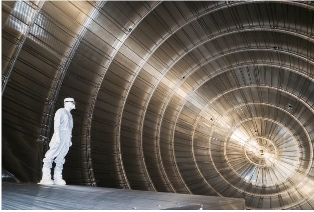
Fig. 2 Wire electrode system inside the KATRIN main spectrometer during installation, photo: M. Zacher.
