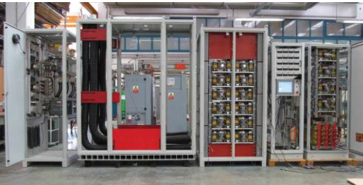
Three new MA acceleration cavities installed (50 kV, h=2 ) and power converters
