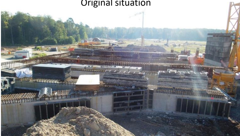
Reinforcement of SIS18 roof and new technical operation building TG1 completed.
