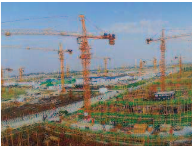
Fig. 1: Construction site of the New Xi'an Jiaotong Research Campus
