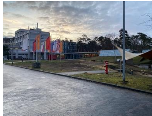
FCC building: Preparatory steps of the FCC site started in March 2021
