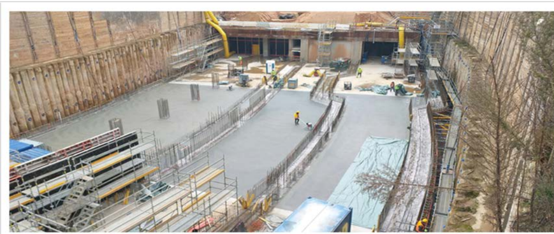
December 2020 SIS100 ring tunnel - ground slab completed
