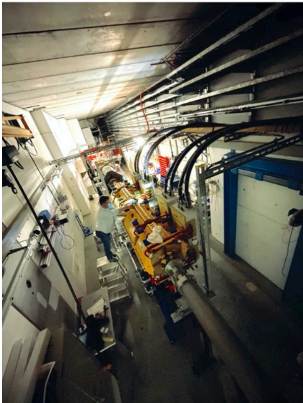
PRIOR-II setup at HHT
