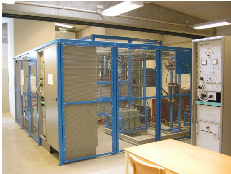
Fig. 3.35. Photograph of dipole power converter (and control cabinet of electron cooler power converter to the left).
