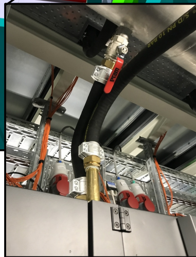
Image: Green Cube ,Data processing centre, GSI Darmstadt KNÜERR DCD Racks, In - & output cooling hoses
