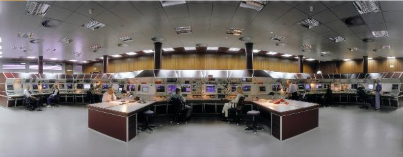
GSI control room (today)
