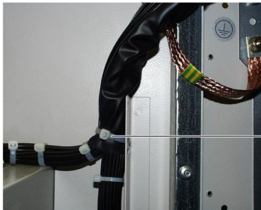
Fig. 65: Cable ties and laying of the protective hose on door
