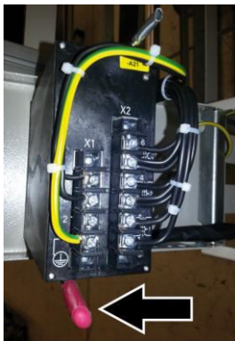
Fig. 33: Protective cap on device protects against injuries on protruding screws.
