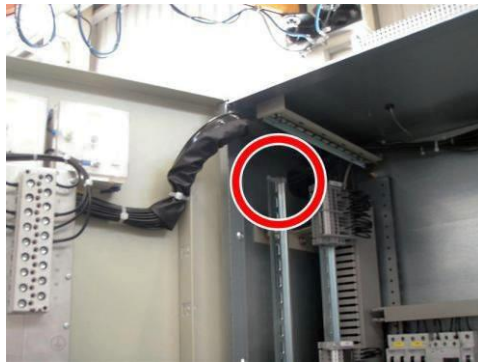
Fig. 6: Avoid sharp edges on mounting rails
