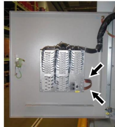
Fig. 17: Ground strap between control/display unit and door
