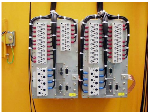
Fig. 54: Cable ties, arranged evenly
