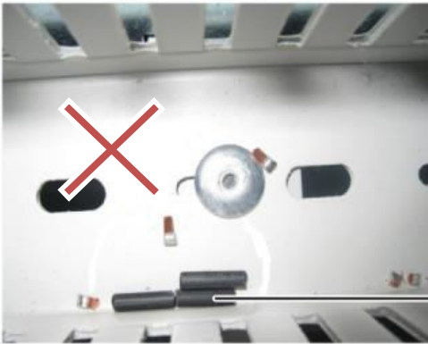
Fig. 85: Falling shavings and residues (1) must not remain in the cabinet and have to be removed with an industrial vacuum cleaner.
