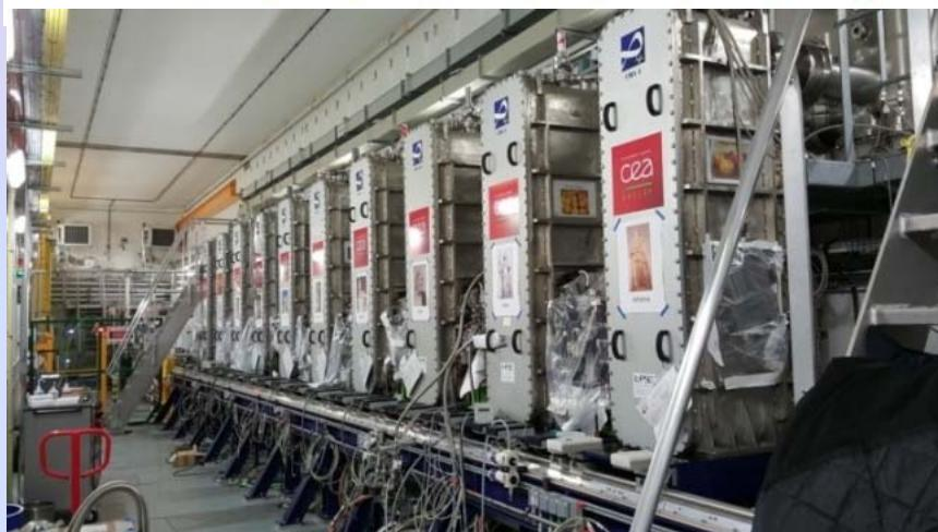
Low  $\beta$  and high  $\beta$  cryomodules installed and connected to their valve boxes.
