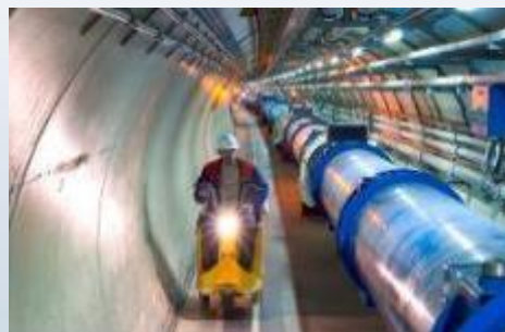
Partial view of the 17 miles-long racetrack
