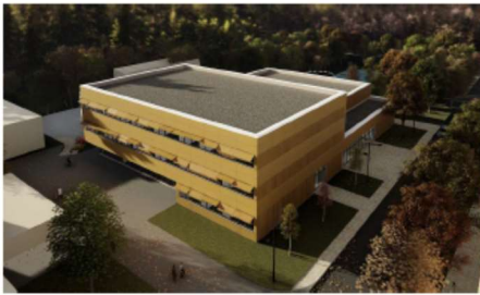
New FAIR control center building at the campus
