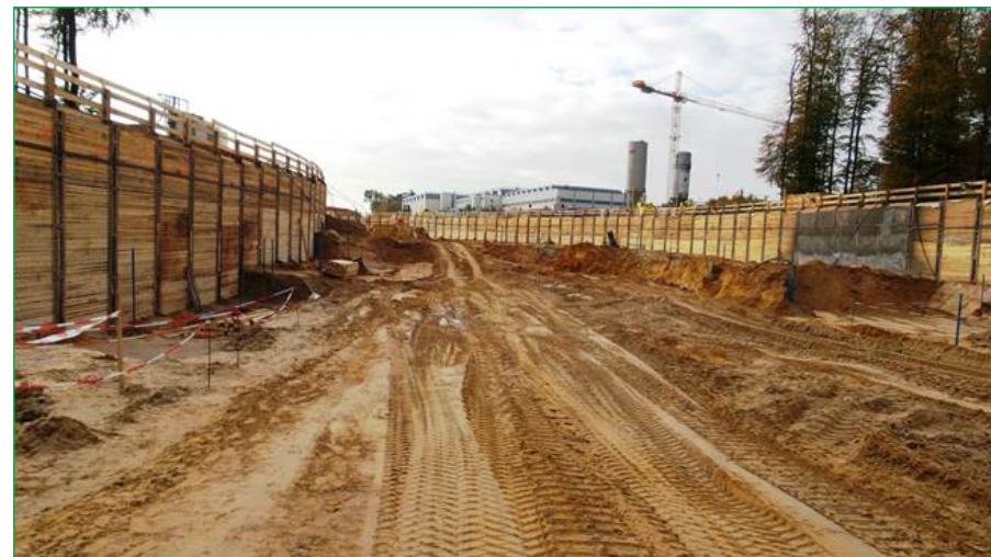
Excavation SIS100 tunnel - Nov 2017
