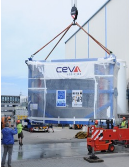
Whole OT in transport frame, 7 \times 5.5 \times 3.5 \text{ m}^3 , 24t, arrival at GSI, Aug. 25, 2023. (Photo courtesy: GSI)
