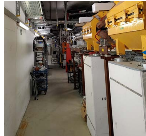
the existing beam line was removed
