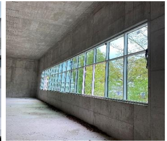
View on the façade in the MCR
