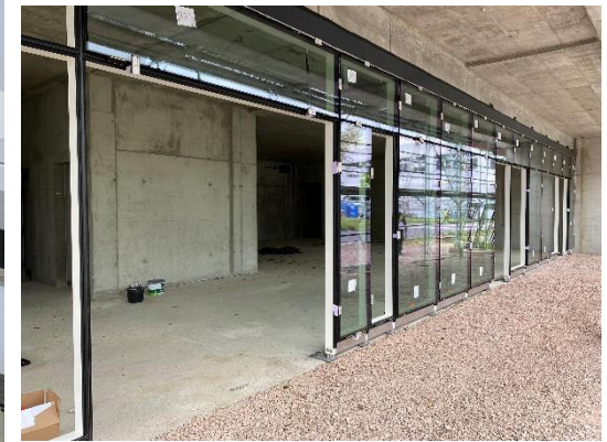
View on the main entrance
