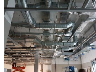
Clean room installation
