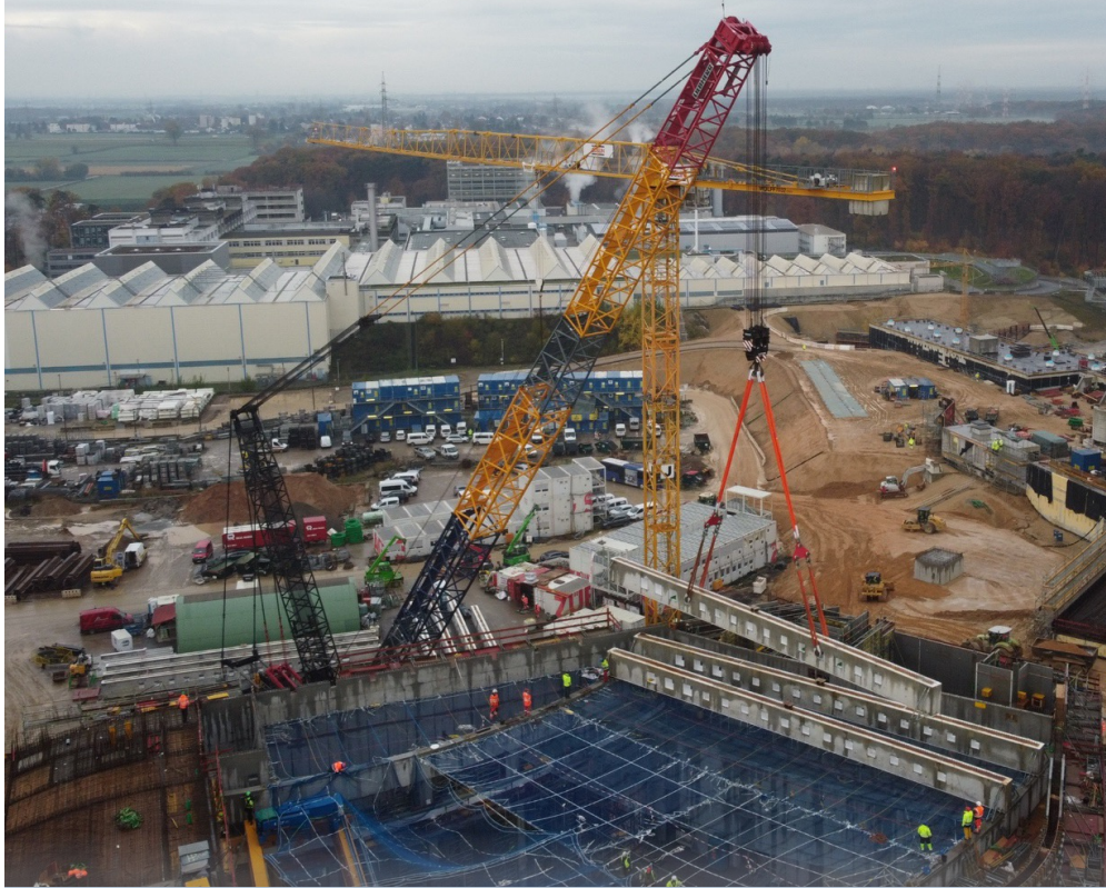
Lifting of the ceiling beams for the roof of the SFRS building "G L0516A".
